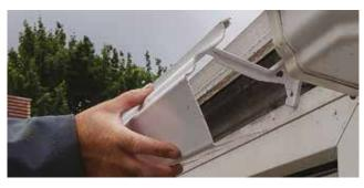
Once front run is fitted to brackets, clip corners to adjoining runs, attach downpipes, and **you've done!**
