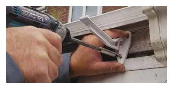
Ensure bracket is vertically aligned and secure with self-drilling screws through two remaining holes.
